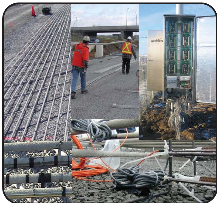
Photos of Highway 40 in Montreal during construction.
