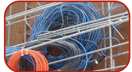
Laurier-Taché Parking Garage SHM system, Hull, QC
