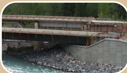
Trout River Bridge, Alaska Highway, BC
