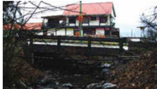
Pont Safe, Duncan, C.-B.
